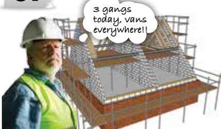
Trusses delivered and lifted into place. Party wall blockwork completed and upper scaffolding removed.
