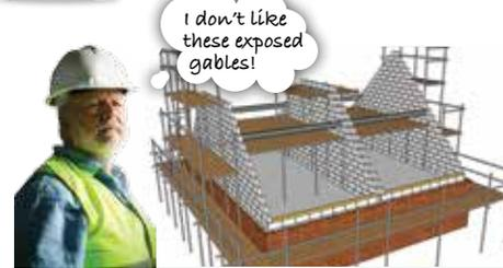
Upper tier scaffolding is built up to allow completion of the gable block work.
